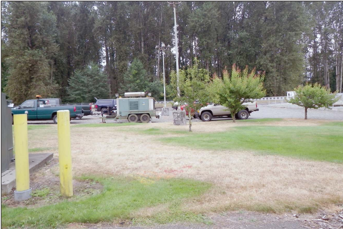
Figure 16. Overview of Area E, looking south.
